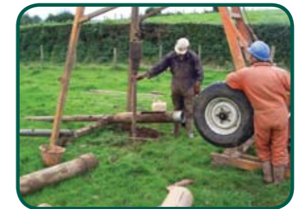
Cable Percussion Drilling
