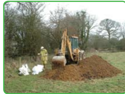
Trial Pit - Hydraulic Excavator
